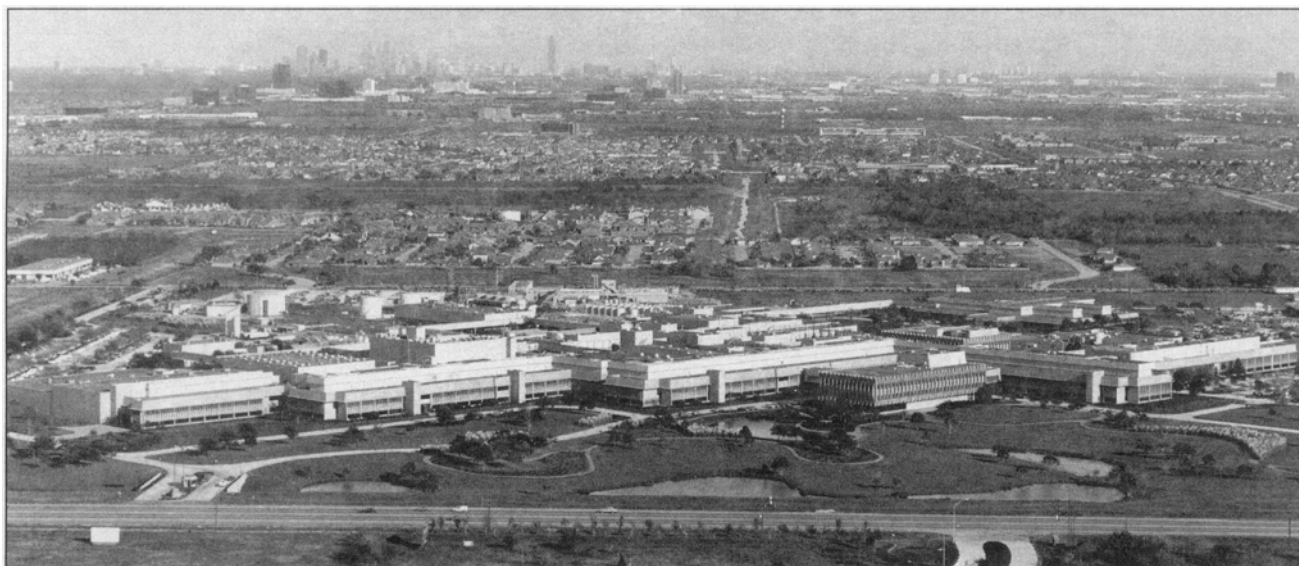
Shell Development Company's Westhollow Research Center, which opened in 1975, occupies 200 acres near Houston, Texas.
